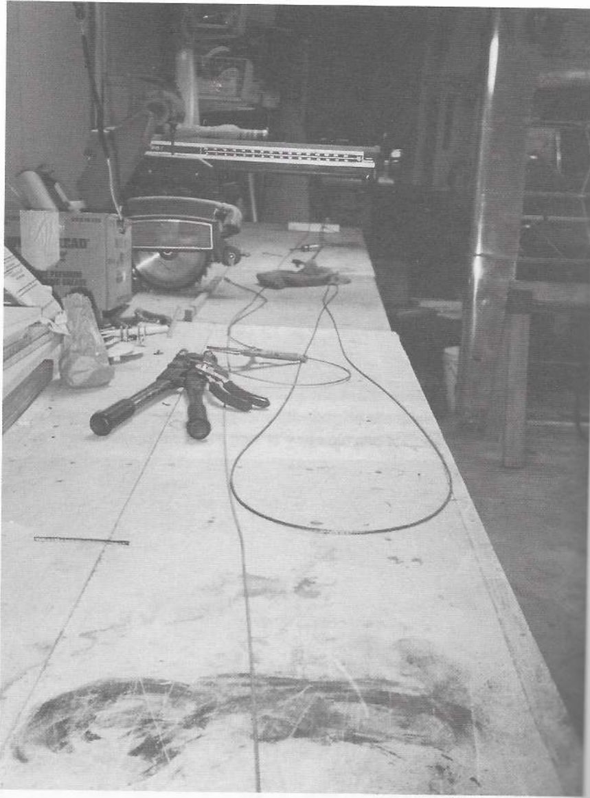
Control cable fabrication . . . all new stainless cables.
